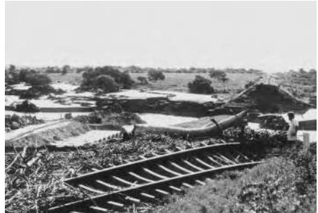
Plate 5 The demolition of a railway line in Swaziland, southern Africa, caused by floods associated with a large tropical cyclone. One role of the applied geomorphologist is to undertake post-event surveys in order to ascertain past discharges
